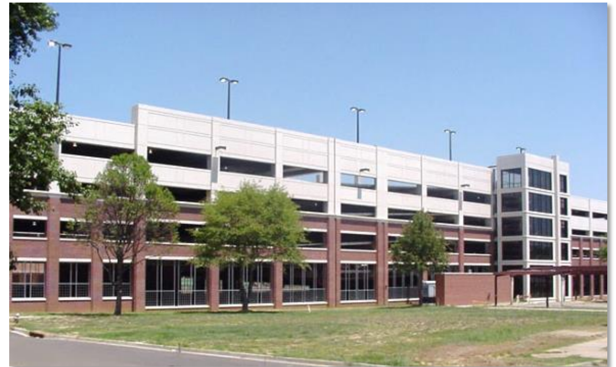
Zach Curlin Parking Garage
