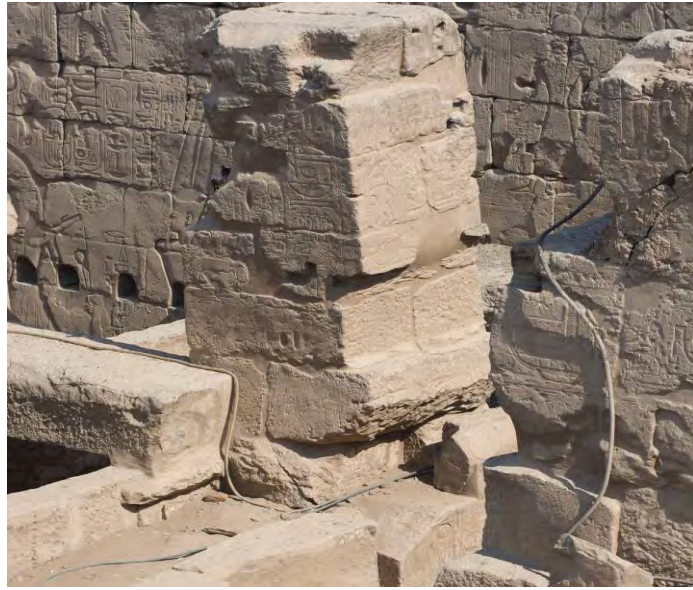
Fig. 3: Rectangular pillar extending above the west wall of the Amun chapel with alterations made to accommodate the raising of the chapel's roof.
